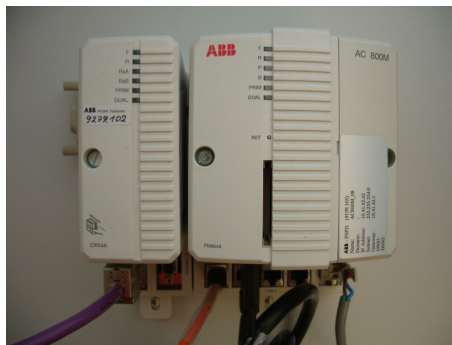
Figure 2.5: Control IT AC800M
