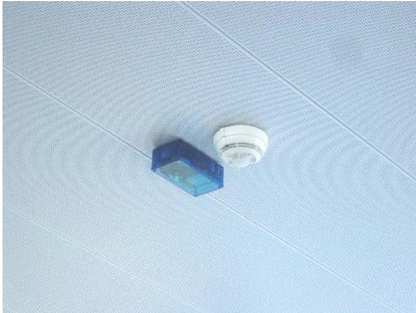
Figure 2-5: "Blue Box" at the ceiling close to a fire detector
