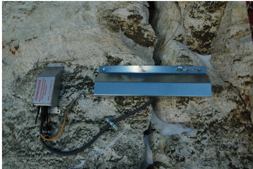
Figure 4-2 Sensornode with attached crack meter (below shielding) and thermistor chain (black cable)
