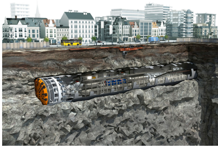
Figure 2.1: A TBM in action 1
